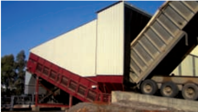
Full Enclosure with Flexible Entry Curtain but without Dust Extraction
