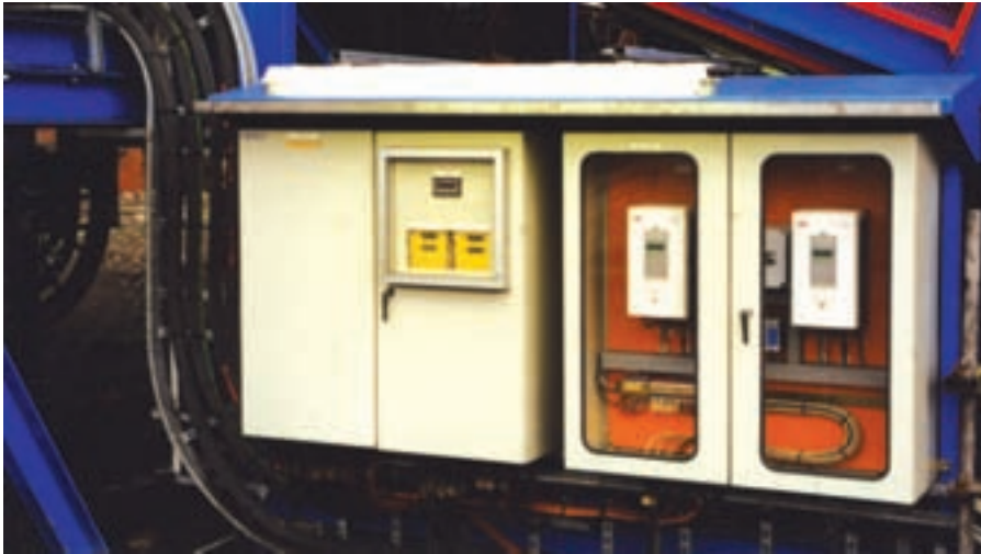
Inverter Speed Control Modules located local to the SAMSON™ but linked to a remote control room
