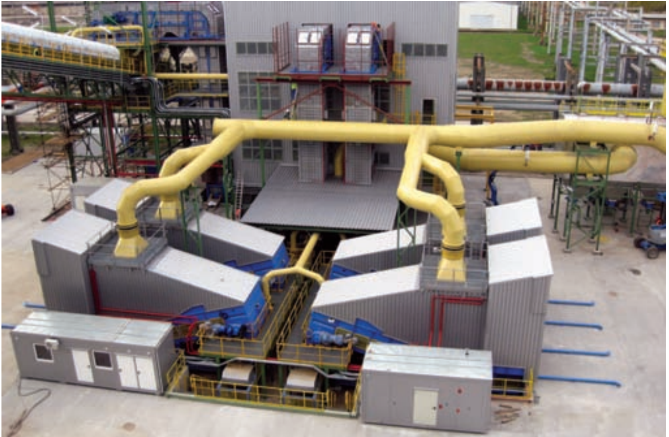
Four SAMSON™ Surface Feeders provide an Alternative Fuel Intake facility to a major Power Plant
