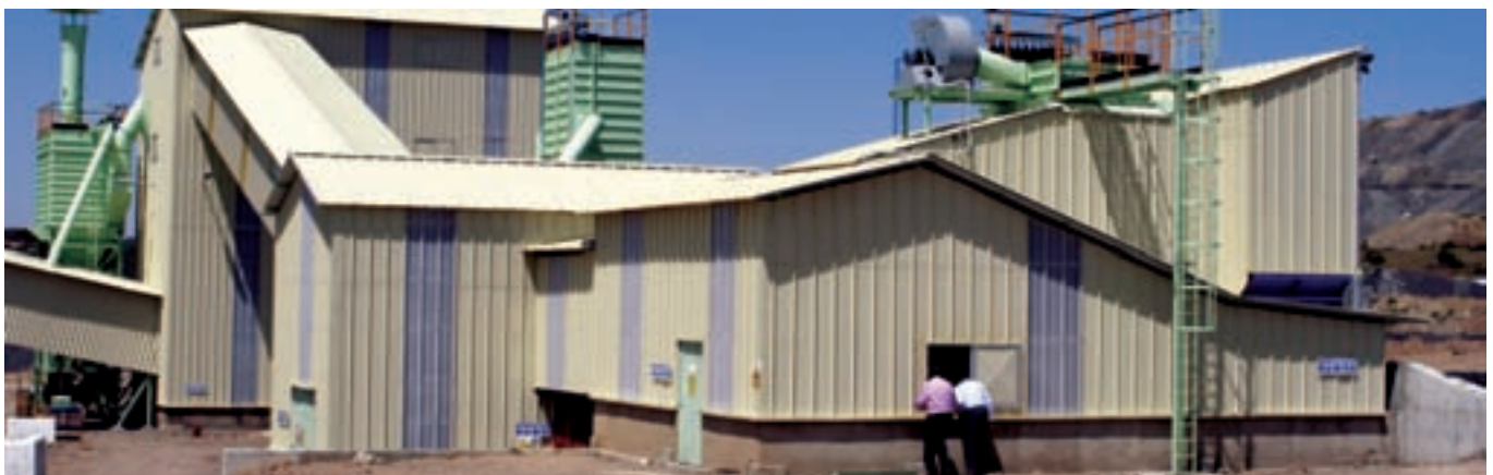
The SAMSON™ enclosure integrated to a complete coal preparation plant handling ROM material direct from the adjacent open cast mine
